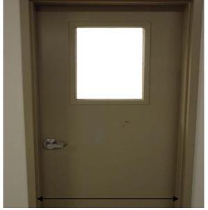
"Measure door stop to door stop for maximum opening" For PLS machines minimum opening required of 40 inches. Note: If your door does not meet above spec please contact your Sales Rep or ULS Support for recommendations. <u>Support@ulsinc.com</u>
